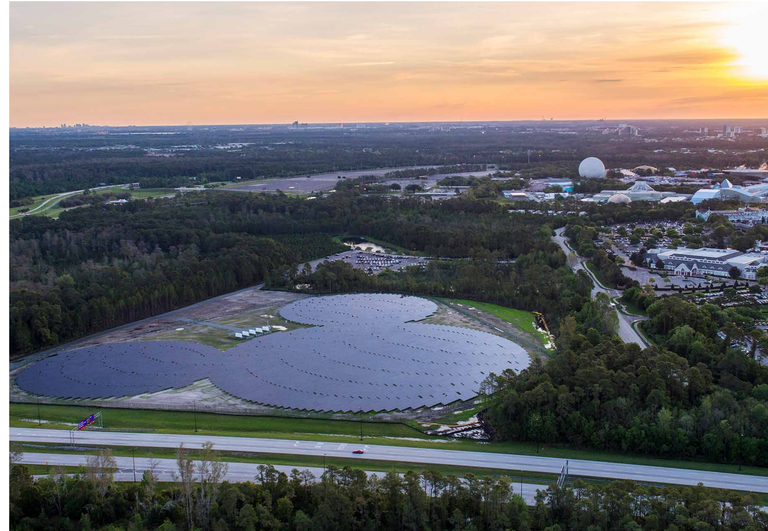
Solar array at Walt Disney World
